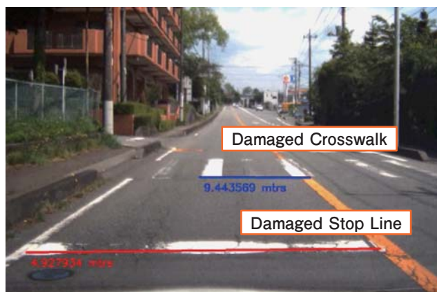
Figure 5 Example of detecting damaged stop line and crosswalk
